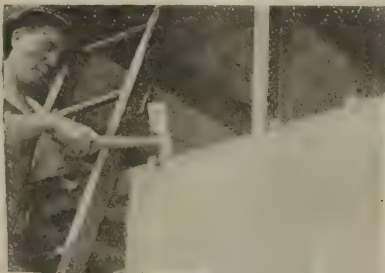
"Close up" of method of attaching slabs to steel work
